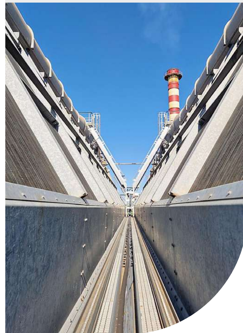
Orion's facility in Ravenna, Italy.
