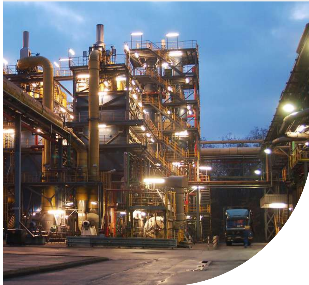
Orion's plant in Cologne, Germany.
